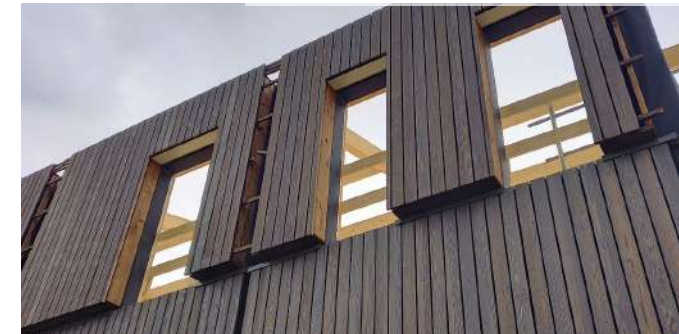
Elévations ossature bois
