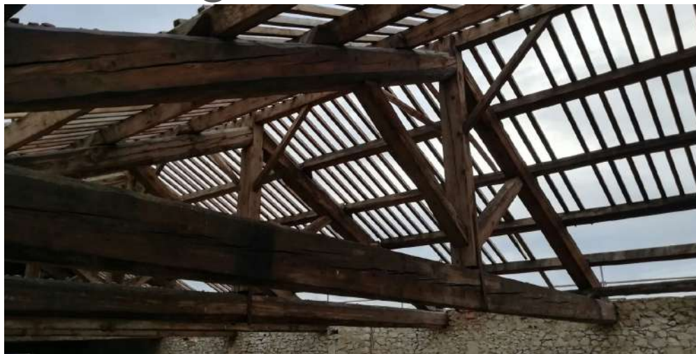
Reprise charpente hangar
