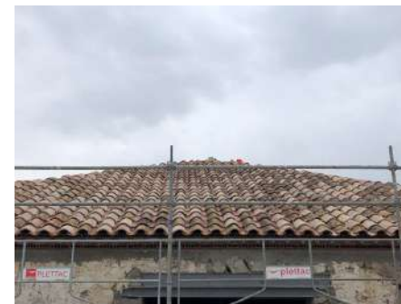
Pose tuile - Hangar
