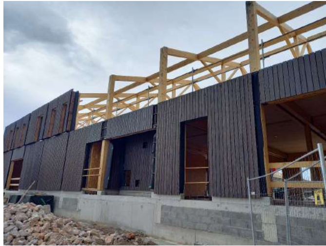
Elévations ossature bois
