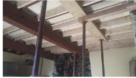
Consolidation plancher
