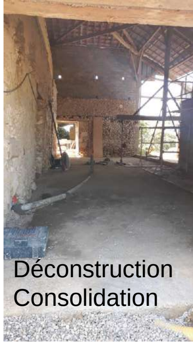
Consolidation plancher
