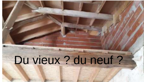
Consolidation plancher
